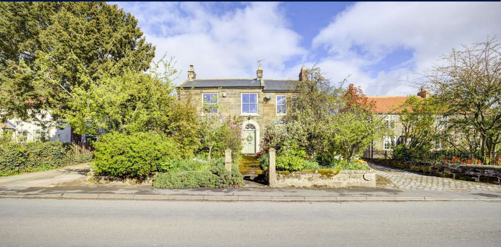
CARLTON HOUSE, EAST HARLSEY, NORTHALLERTON NORTH YORKSHIRE, DL6 2DB
