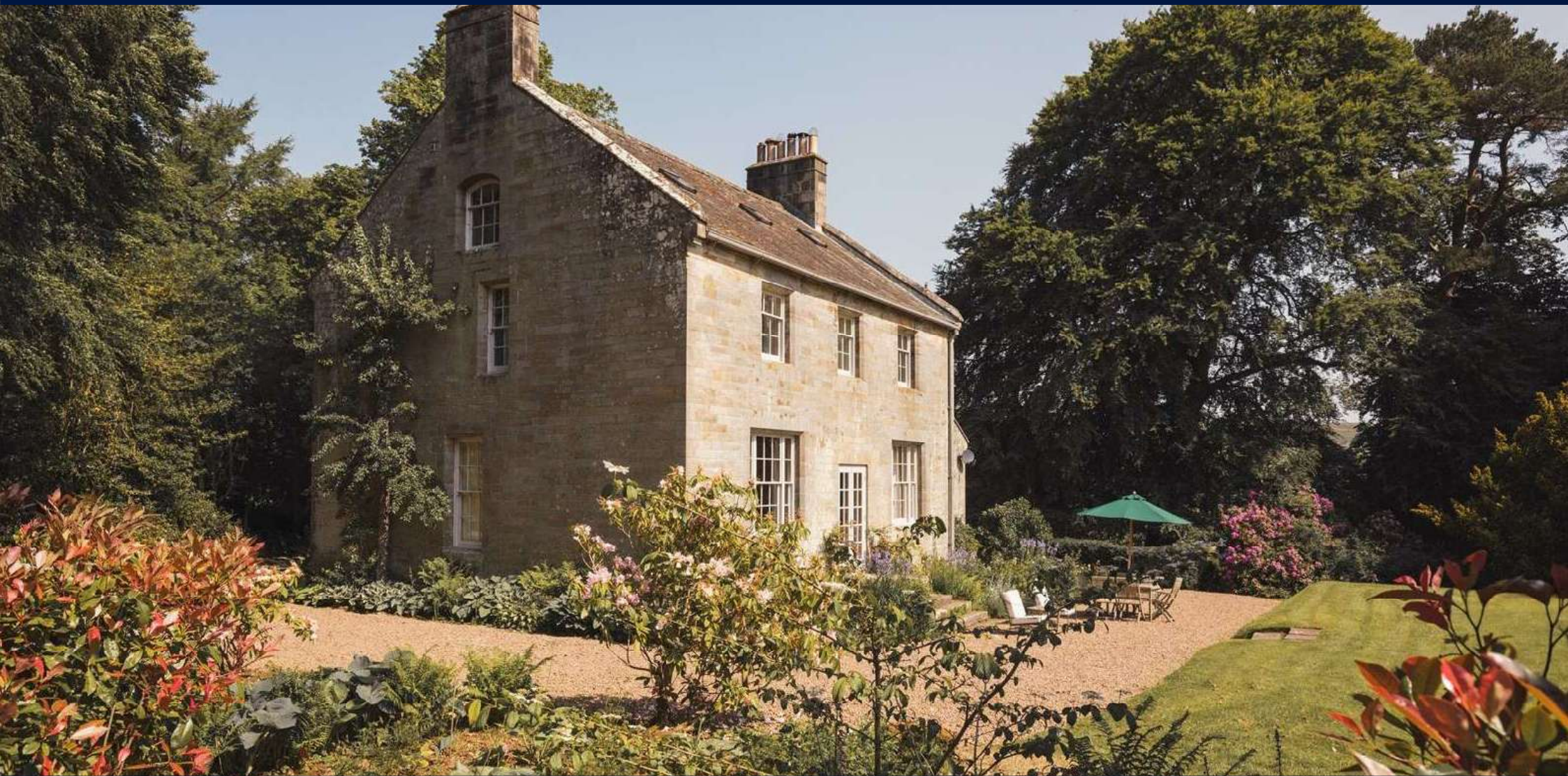
GREYSTEAD RECTORY AND COTTAGE, TARSET, HEXHAM, NORTHUMBERLAND, NE48 1LE
