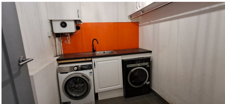
Wall and base units, plumbing for washing machine, radiator
