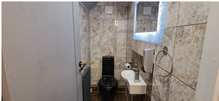
Low flush WC, hand wash basin, tiled floor and walls.
