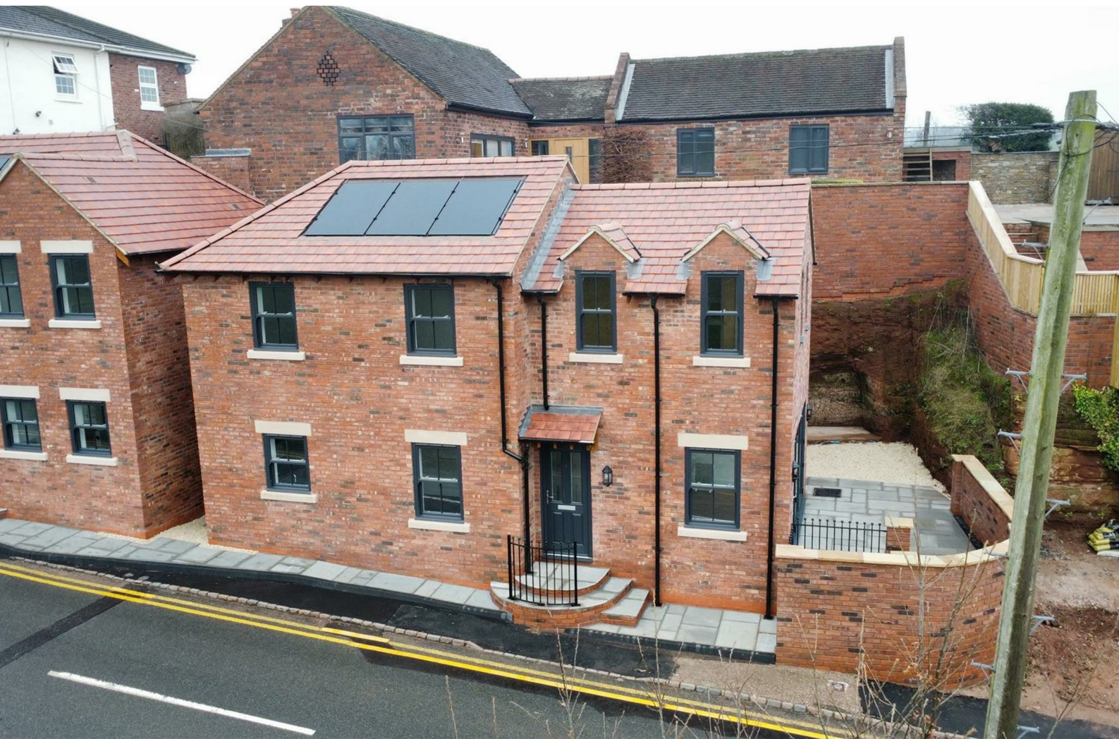
Tavern Cottage Caunsall Road, Cookley DY11 5YH
