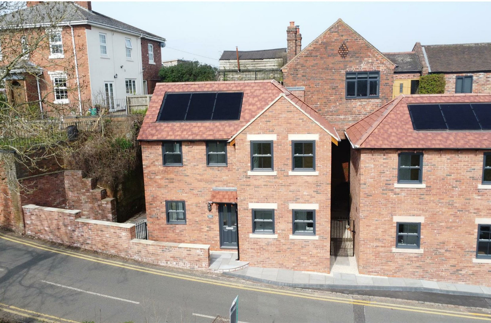
Sandstone Cottage Caunsall Road, Kidderminster DY11 5YH
